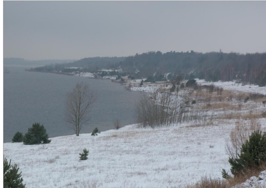
Length of the affected area ~ 1.500 m
