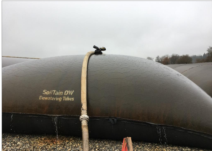
Dewatering tube in action (15 m circumference by a length of 35 m)
