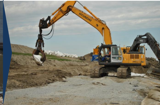
Installation by a backhoe with a modified grab
