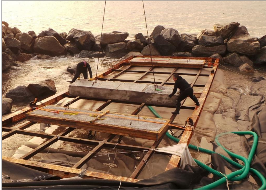
Installation frame to keep the unfilled tube in place
