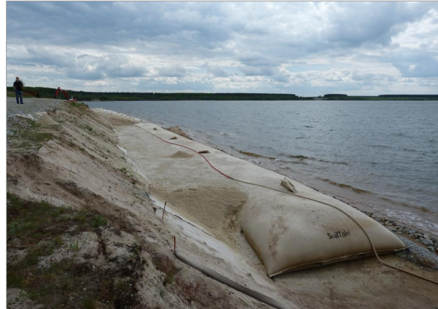
Backfilling of the area after successful first layer installation
