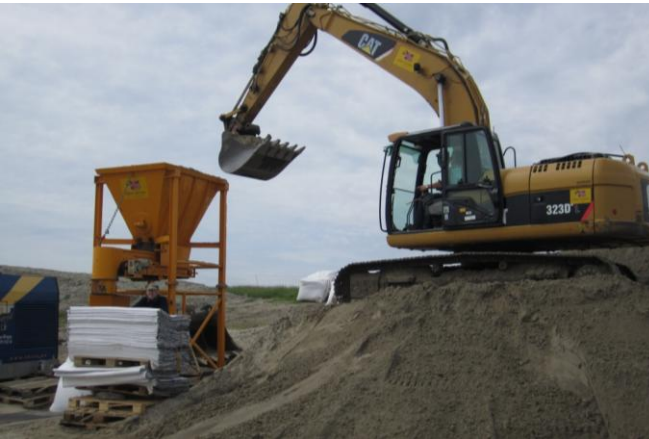
Filling by use of a funnel and a backhoe
