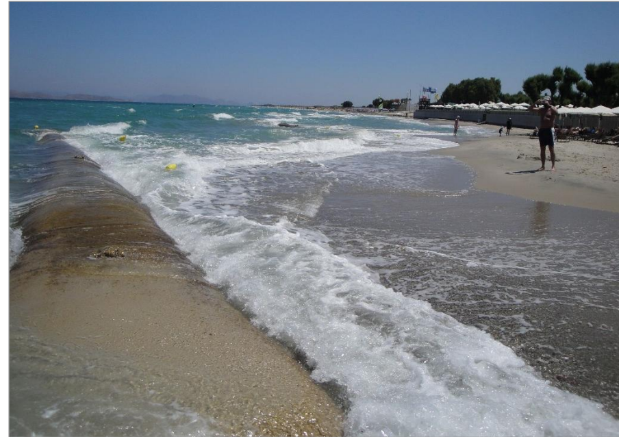
Kos Island, Neptune Beach Resort, 2015 after installation
