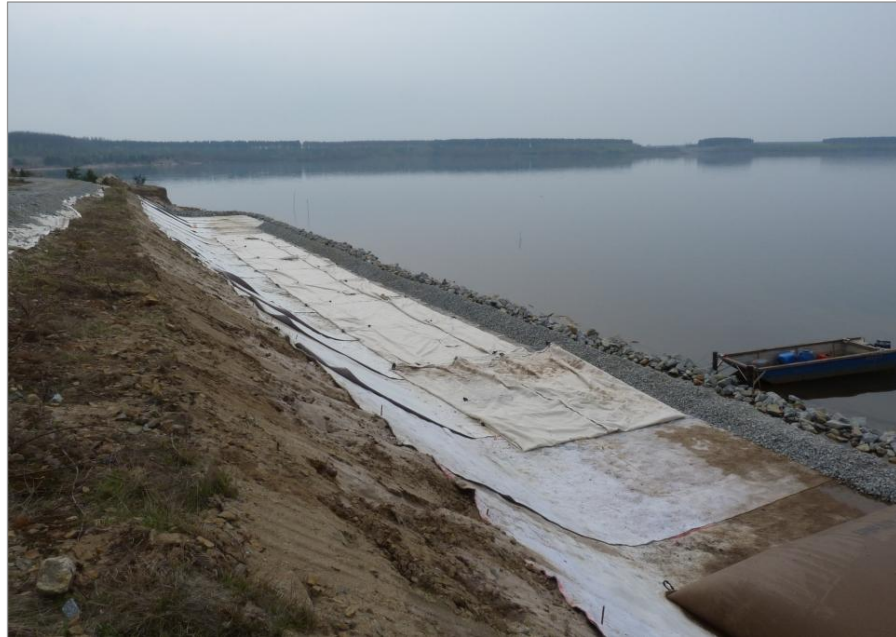
Lay out of the empty tube on the prepared platform
