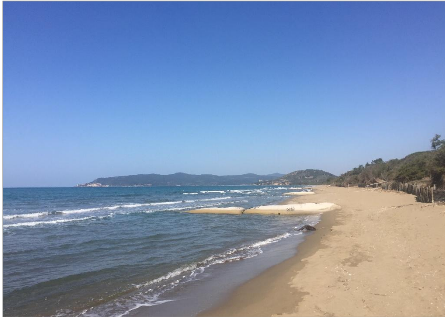
SoilTain CP tube Diameter=1.5m
